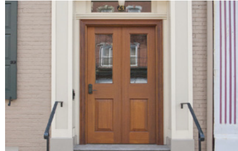
Modified historic door to allow for a wider opening while maintaining the appearance of a paired door
