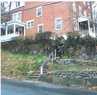
Multi-level stone retaining wall
