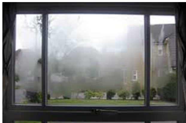
Window with condensation due to faulty gasket seal
