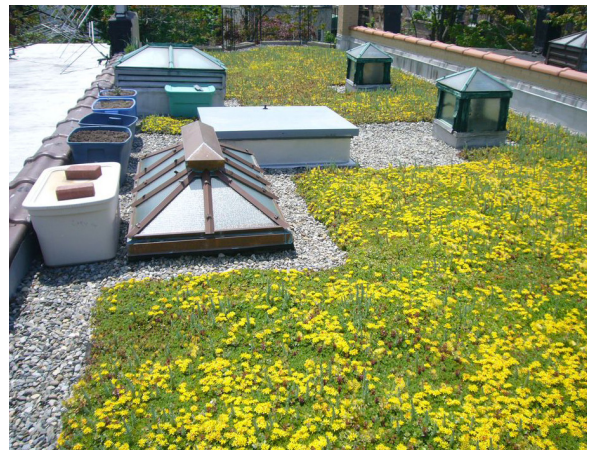
Green roof on a historic building flat roof Source: iGrownews
