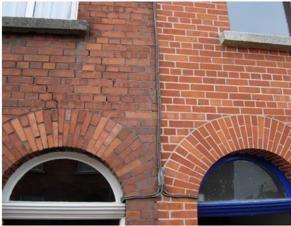
Before (left) and after (right) repointing and cleaning of historic brick
