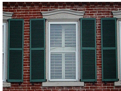
Historic window with wood louvered shutters, wood blinds, and exterior storm windows
