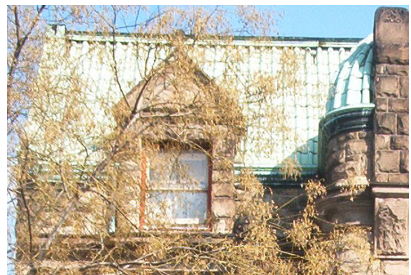
Historic oxidized copper roofing shingles
