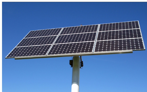
Ground mounted solar panel
