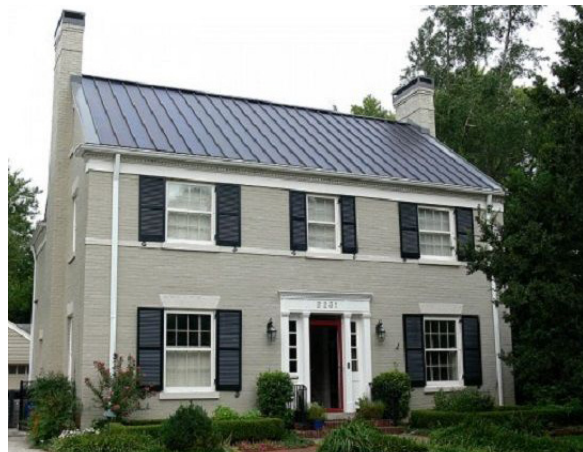
Thin film solar panel system on a 1930s house with a standing seam metal roof
