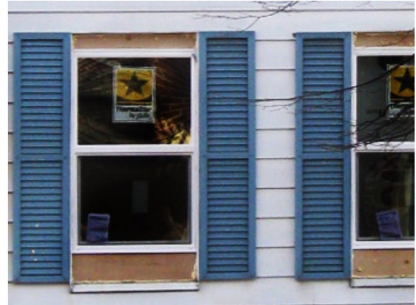
Historic windows inappropriately infilled and replaced with vinyl sash windows. These windows do not have trim and lack the depth of historic wood windows.
