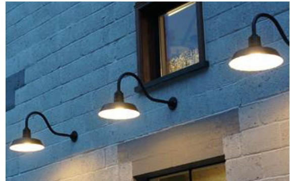
Gooseneck fixtures where the conduit and mounting connections have been concealed
