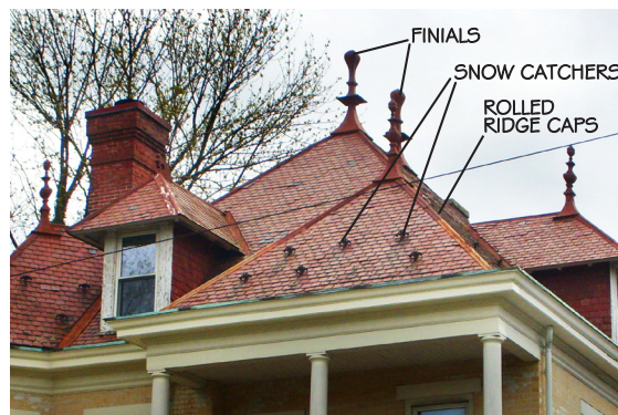
Red slate roof with rolled ridge caps, finials and snow catchers
