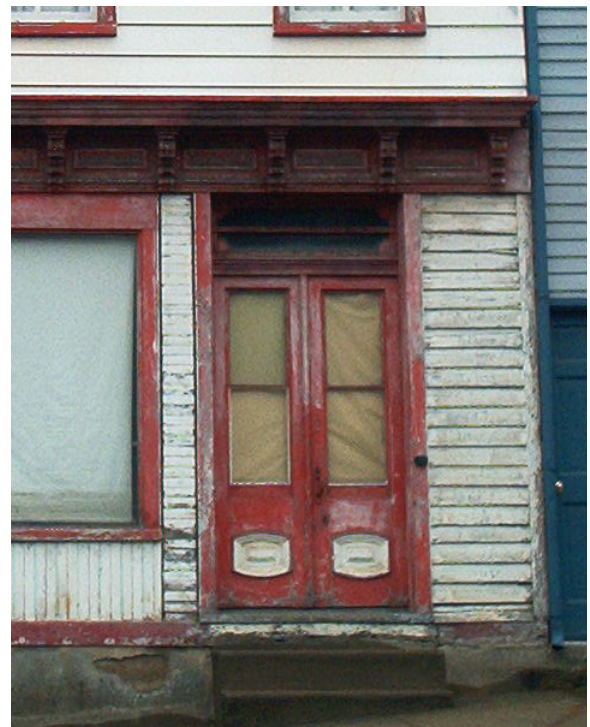
Wood rot and peeling paint are common issues. Minor repair and maintenance can prolong the serviceable life of most historic wood doors.
