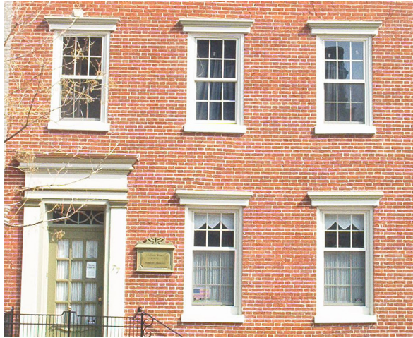
Historic 6 over 6 (second floor) and 6 over 9 (ground floor) multi-light, double-hung windows
