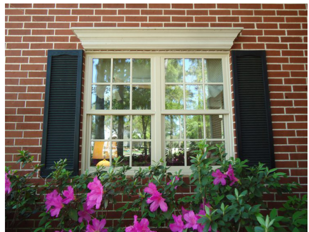
Simulated divided lights in a 6 over 6 window
