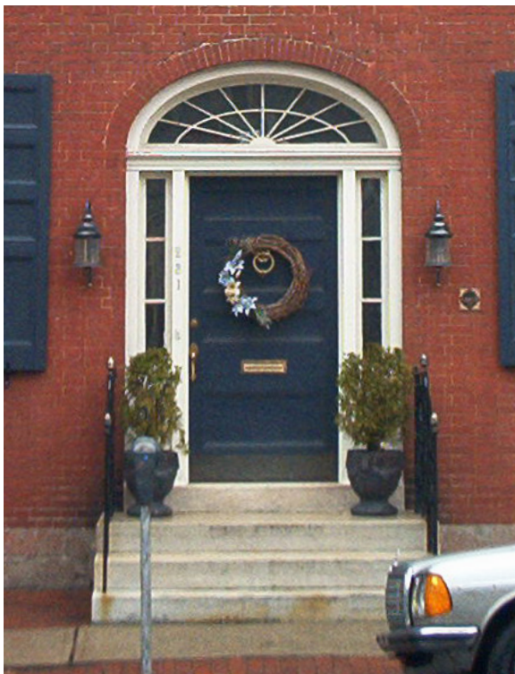
Wood-paneled door featuring a wood surround and decorative arched transom with sidelights on Spring St.
