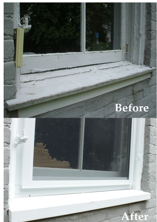
Deteriorated window before and after repair, repainting, and installation of a storm window
