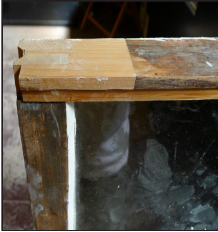
Historic wood window with replaced 'Dutchman' and new glazing putty. An advantage of historic windows over modern units is easy repairability.
