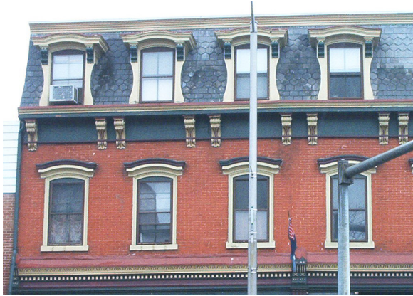
Slat shingle Mansard roof on Northampton Street
