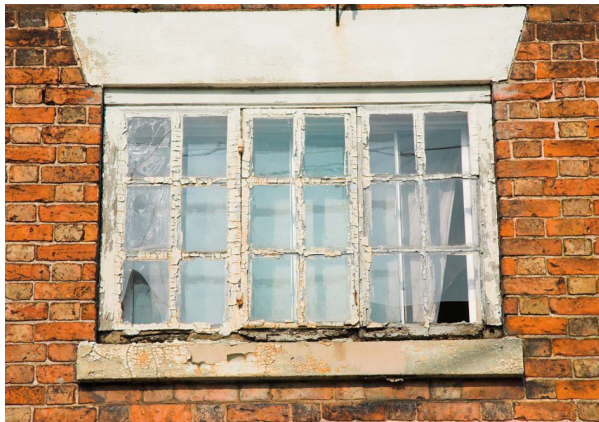
Deterioration typically starts at the sill. Peeling paint allows in moisture which causes the wood to rot.
