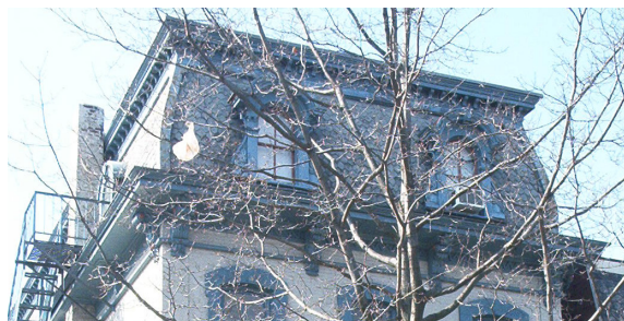
A Mansard roof with slate shingles and dormers
