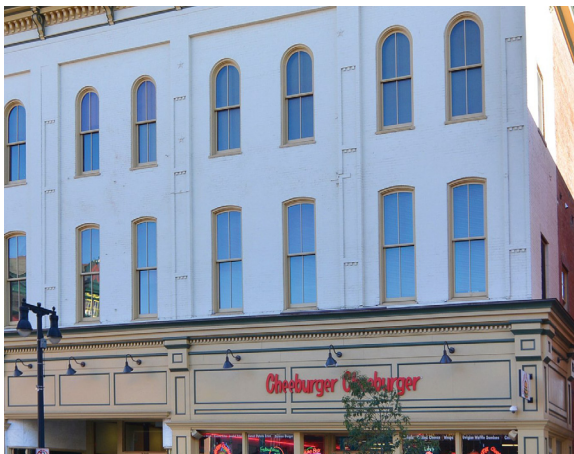
Replaced double-hung windows with insulated glazing at the Pomeroy Building in Easton
