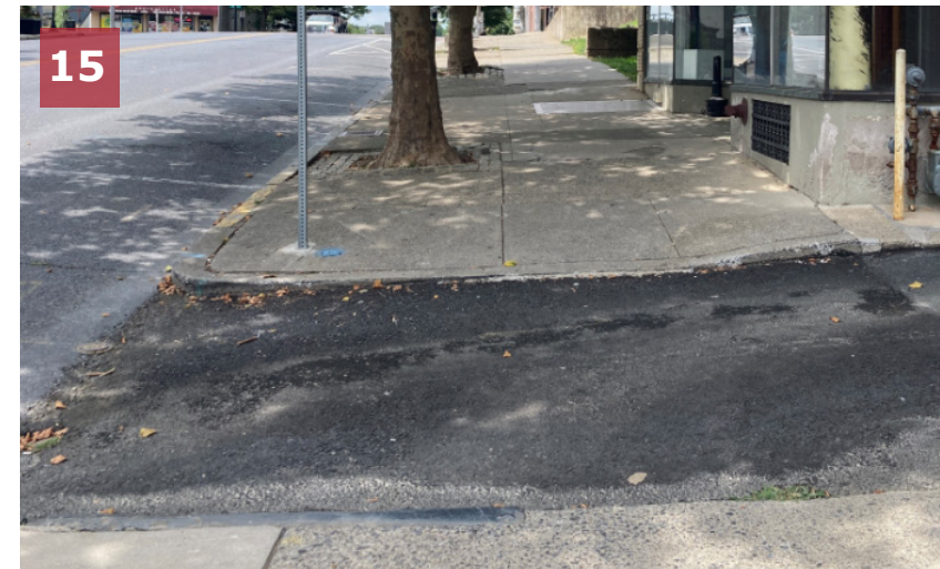
Missing curb ramps at the intersection of Northampton Street & Library Court (two corners).
