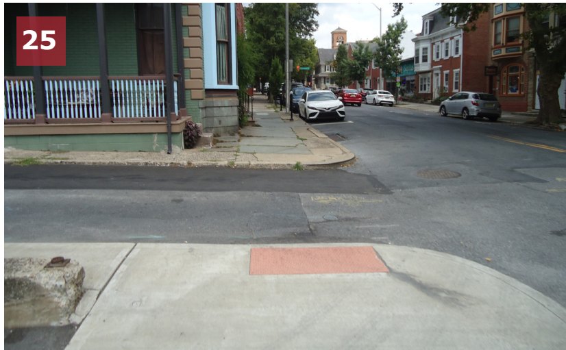
Non-compliant curb ramp at the intersection of Second Street & Pine Street (four corners).
