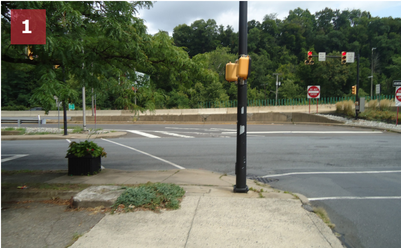
Non-compliant curb ramps at the intersection of Fourth Street & Bushkill Street (four corners).
