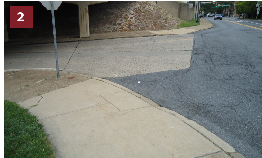
Missing curb ramps at the intersection of Bushkill Street & Bank Street (four corners).
