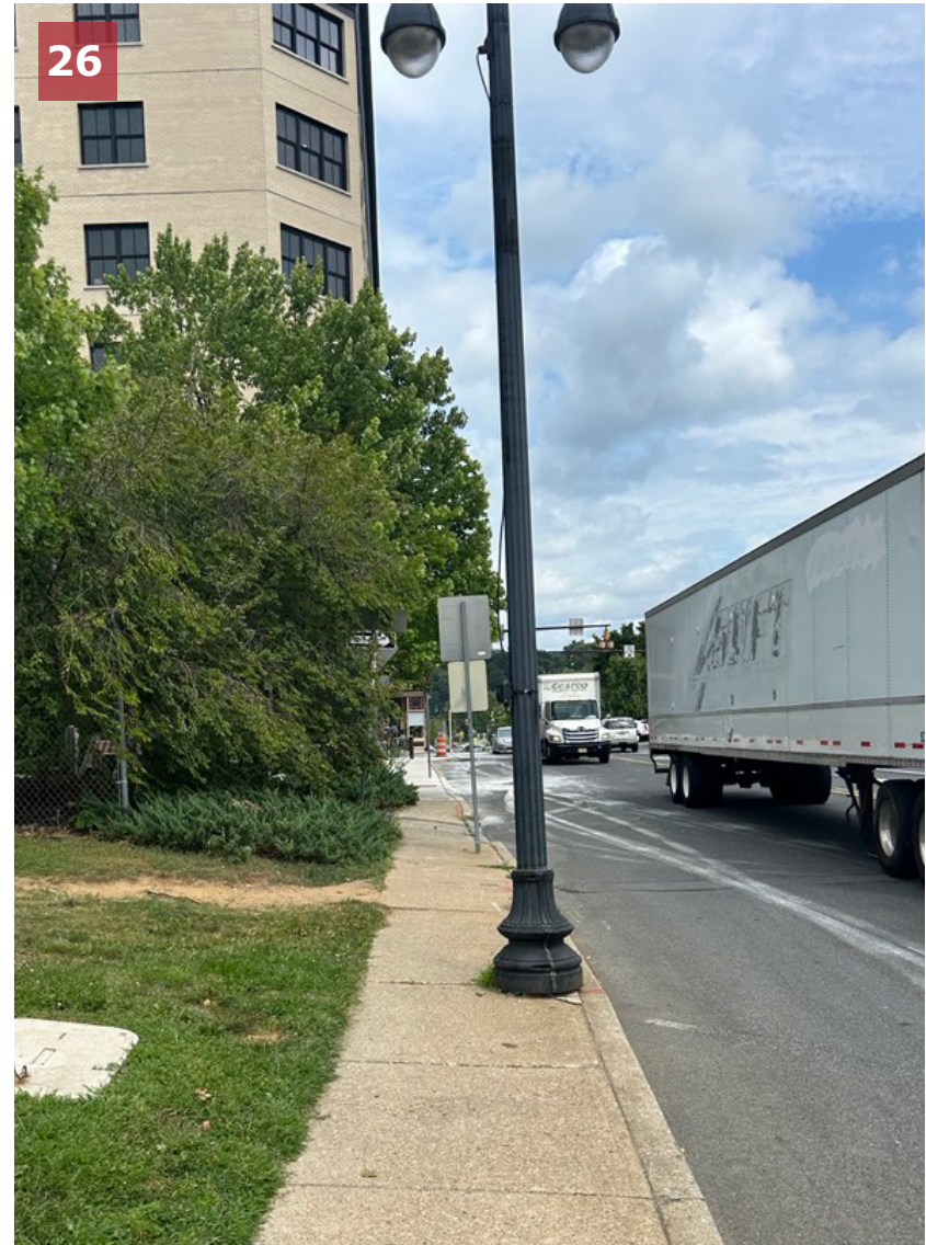
The lamp posts and street signs limit the pedestrian access route along the west side of Larry Holmes Drive.
