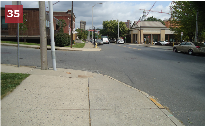
Missing/non-compliant curb ramps at the intersection of S. Fourth Street & Michael J. Koury Place (two corners).
