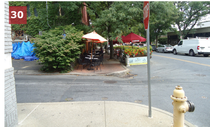
Missing curb ramps at the intersection of Ferry Street & Sitgreaves Street (four corners).
