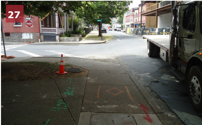
Missing/non-compliant curb ramps at the intersection of Ferry Street & Bank Street (two corners).
