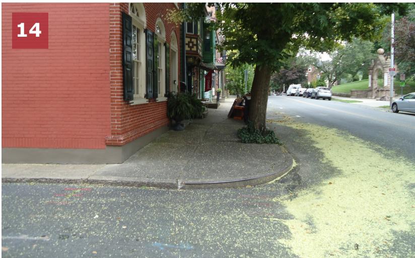
Missing curb ramps at the intersection of Second Street & Church Street (four corners).
