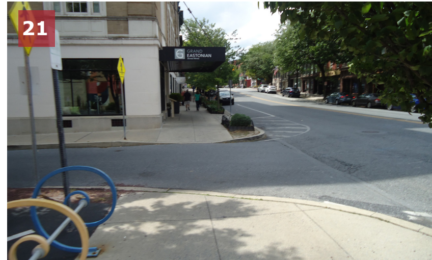
Missing curb ramps at the intersection of Northampton Street & Green Street (two corners).
