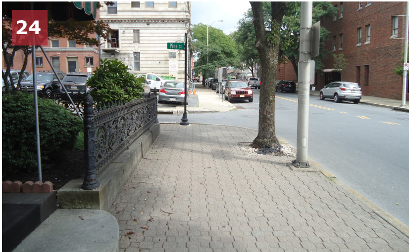
Missing/non-compliant curb ramps at the intersection of Fourth Street & Pine Street (four corners).
