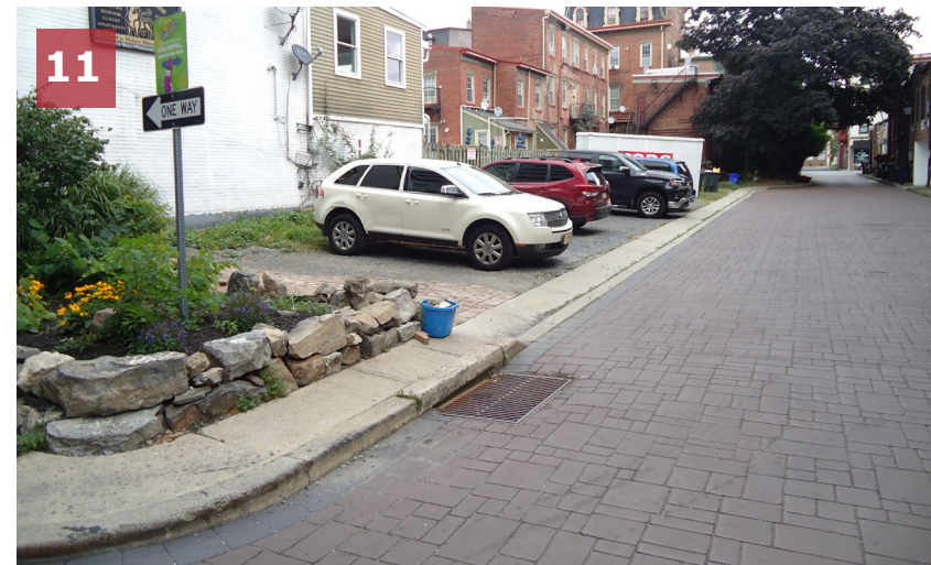
The sidewalk on the north side of Church Street between Bank Street and Third Street is narrow, has a significant cross slope, and does not have curb ramps.
