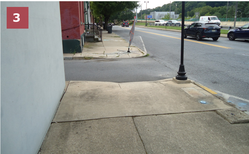
Non-compliant curb ramps at the intersection of Bushkill Street & Green Street (two corners).
