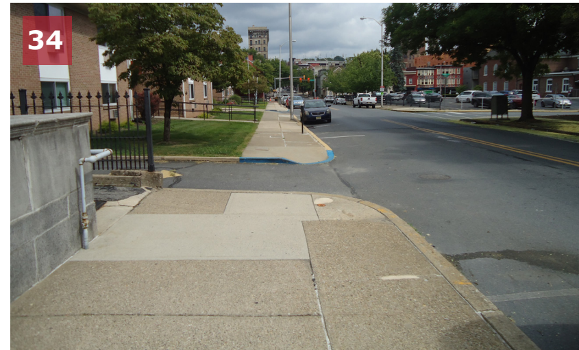
Missing/non-compliant curb ramps at driveway to Fourth Street (two corners).
