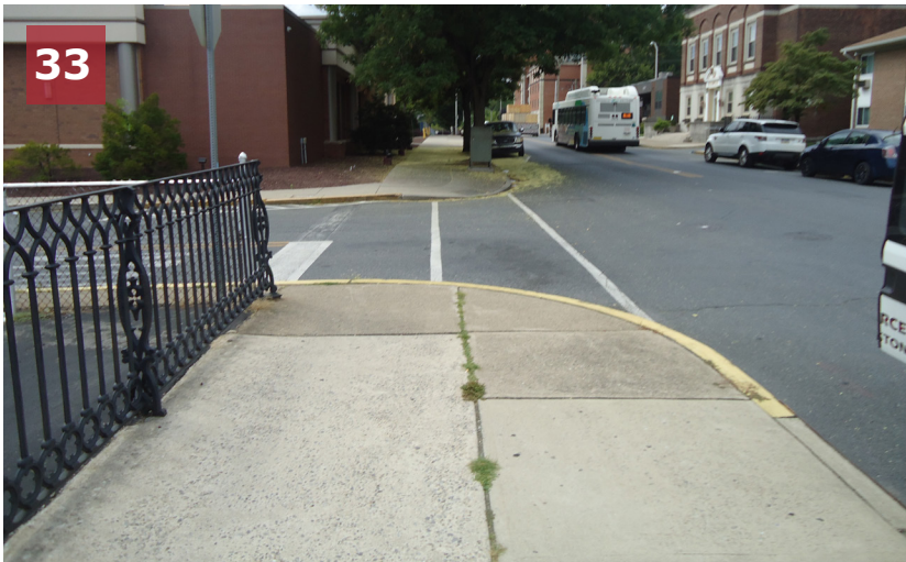
Missing curb ramp at the intersection of Fourth Street & Spruce Street (one corner).
