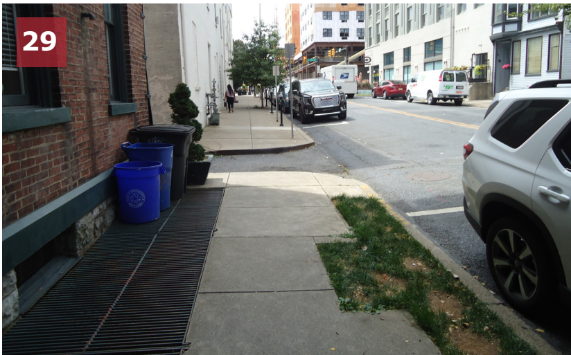
Missing curb ramps on south side of Ferry Street (two corners).
