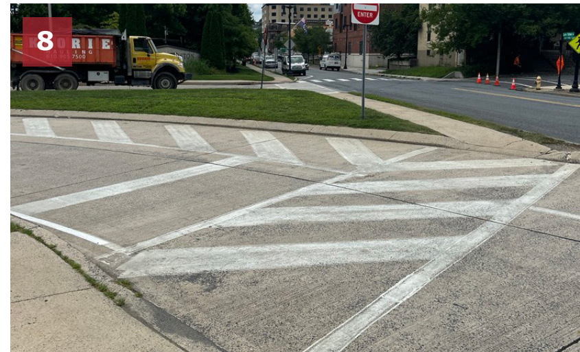
Non-compliant curb ramps at the intersection of Larry Holmes Drive & Route 611 (four corners)
