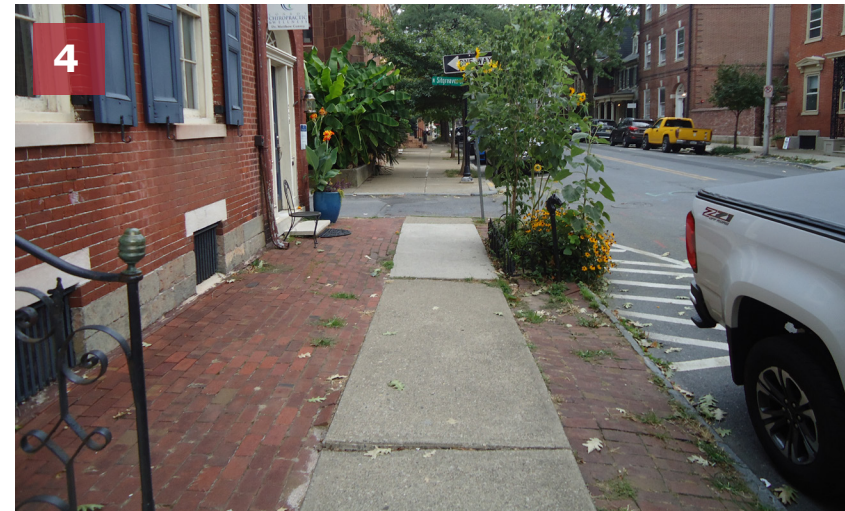
Missing curb ramps at the intersection of Spring Garden Street & Sitgreaves Street (three corners).
