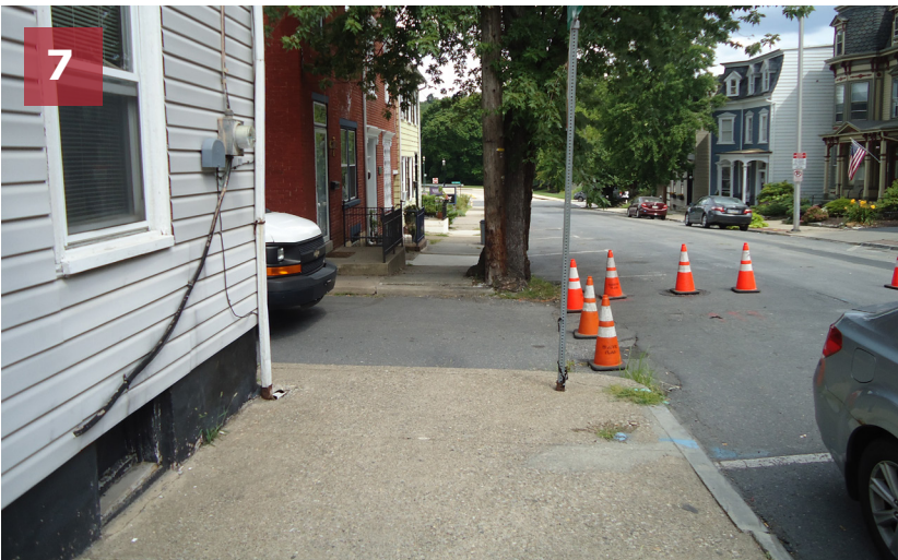
Missing curb ramps at the intersection of Spring Garden Street & Green Street (two corners).
